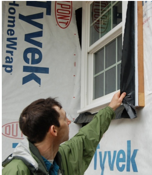
Figure 17. Windows built-out for exterior foam insulation
