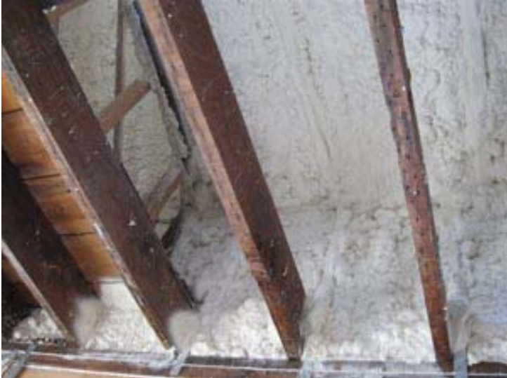
Figure 21. Spray foam under front bay window
