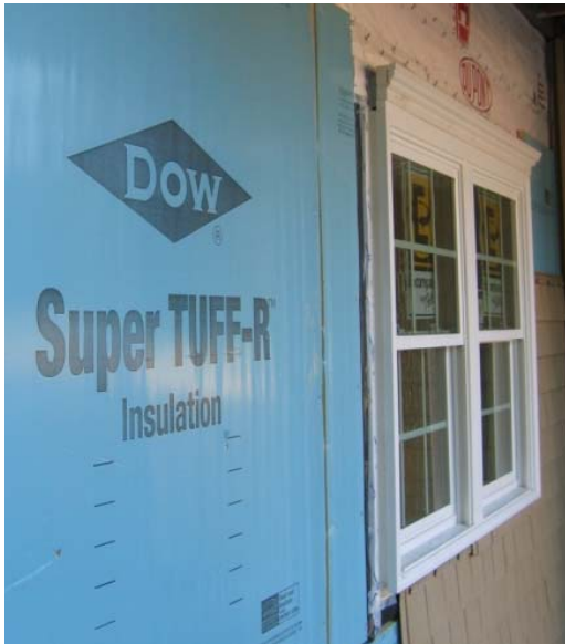
Figure 6. Windows are built out to accommodate the exterior rigid foam insulation
