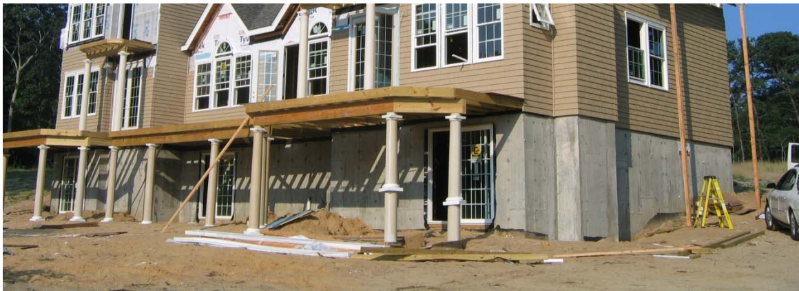
Figure 8. Walk out basement
