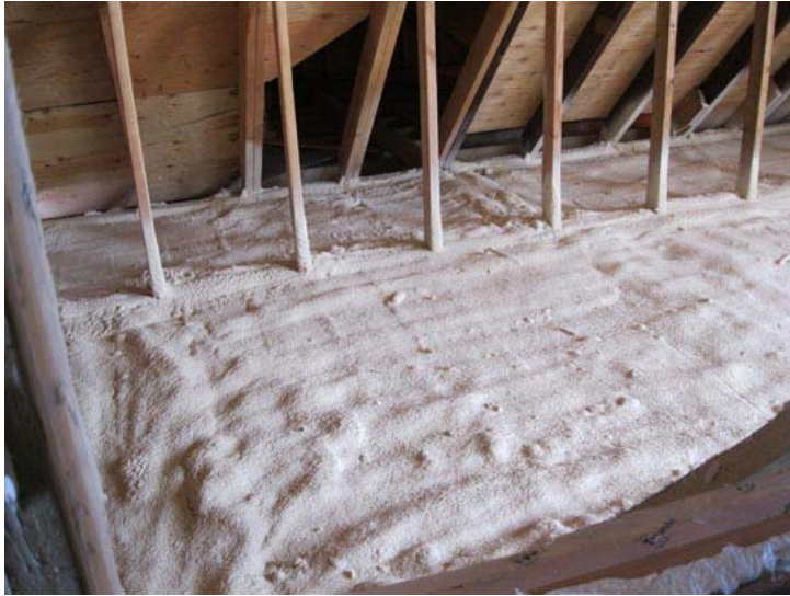
Figure 19. Spray foam on the attic floor prior to covering with cellulose
