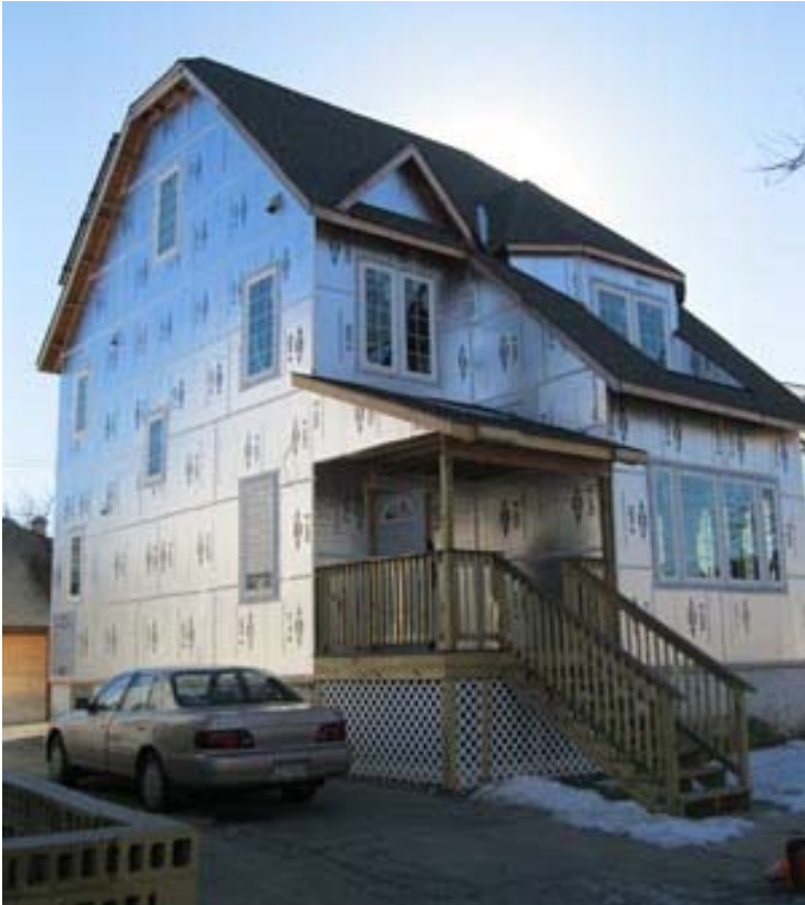
Figure 22. Exterior insulation completed with seams taped
