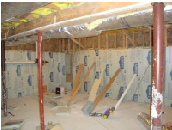
Figure 16. Basement walls with interior rigid foam installed (2" XPS)
