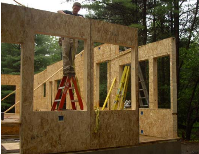
Figure 11. SIPs are 6.5" thick with a polyisocyanurate core, obtaining a total R value of 40
