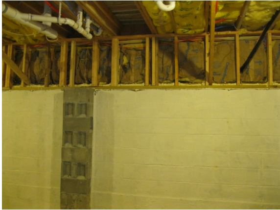
Figure 15. Basement walls prior to installation of interior rigid foam
