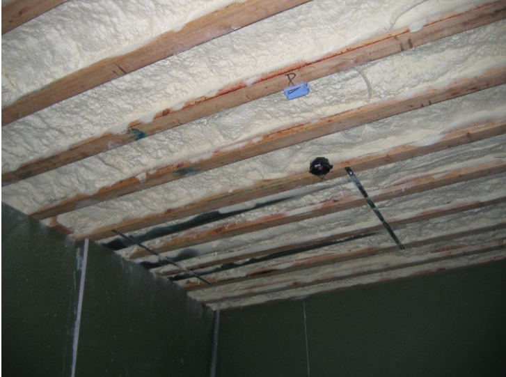
Figure 26. High density spray foam in the garage ceiling
