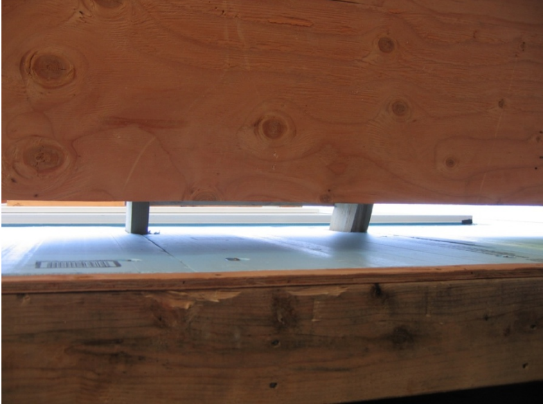
Figure 27. Porch roof (top of photo) is built out from front wall to permit continuous foam insulation and brick to pass behind
