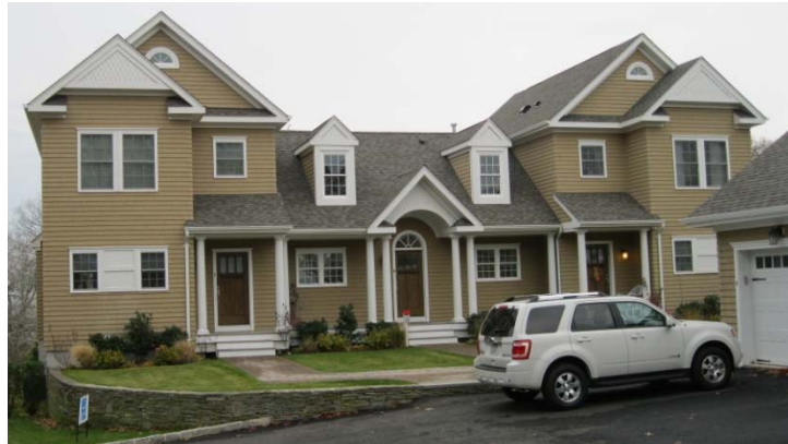
Figure B1: The residence in Hampton Bays, NY; the unit is on the left
