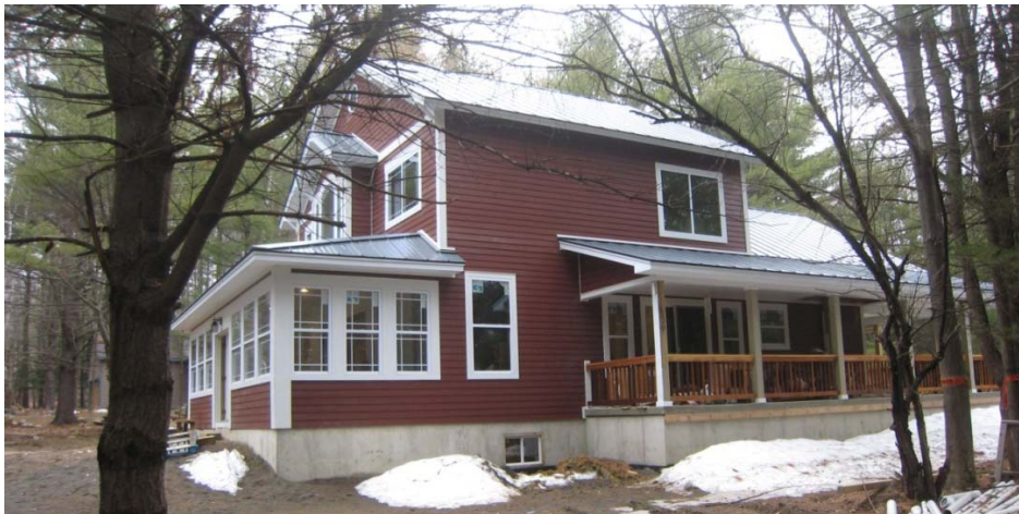
Figure 10. The Stephens House
