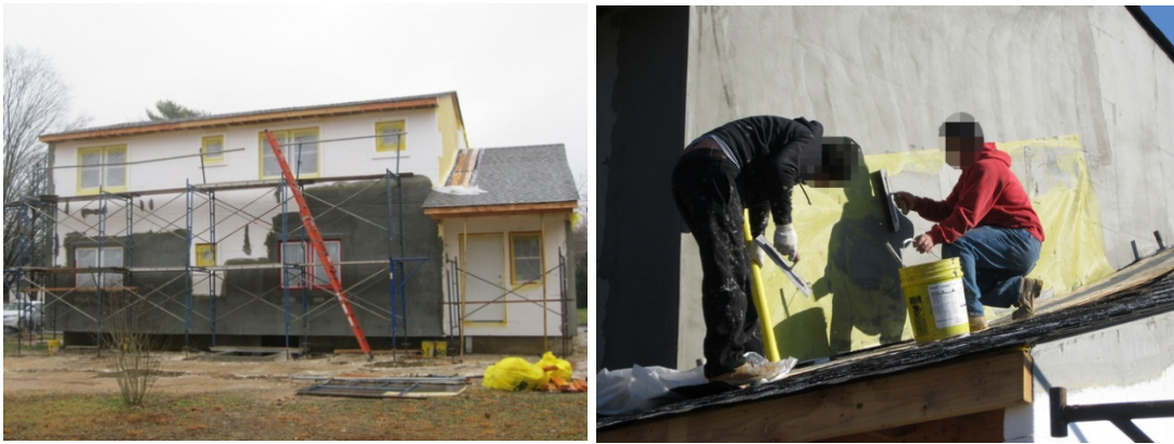
Figure 9. The gray basecoat is troweled on over an embedded layer of reinforcing mesh.
