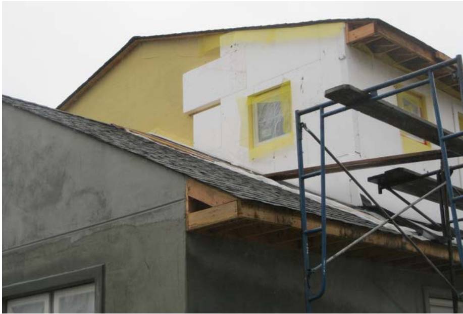
Figure 2. Field-applied EIFS showing yellow water resistive barrier, white EPS insulation with yellow reinforcing mesh, and gray basecoat in foreground
