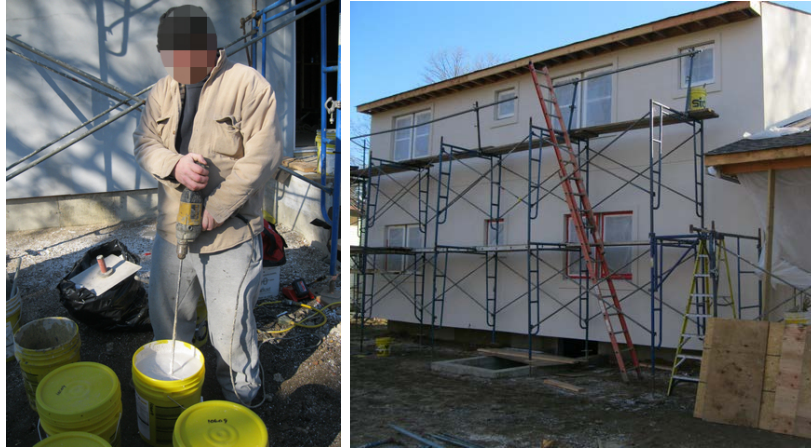
Figure 11. The finish coat is mixed and applied with trowels.
