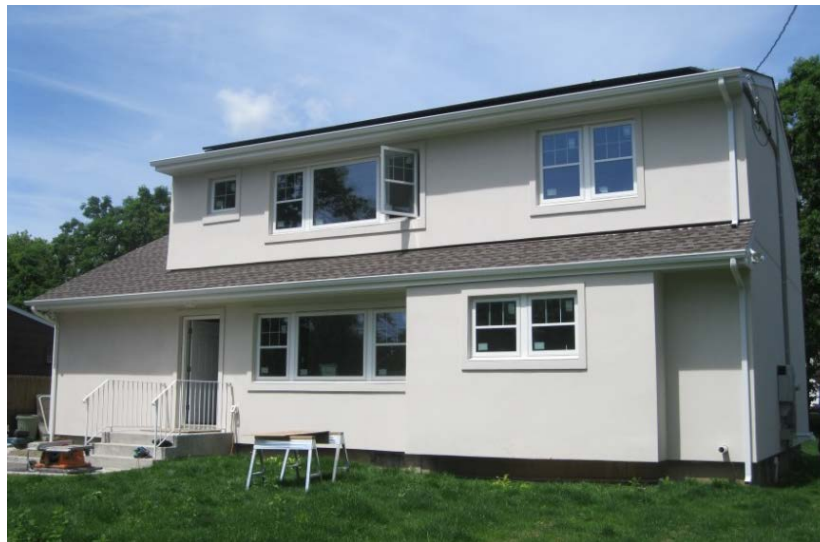
Figure 12. The finished system
