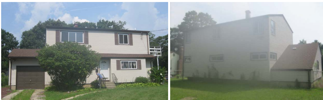
Figure 3. Front and rear elevations of the pre-retrofit home
